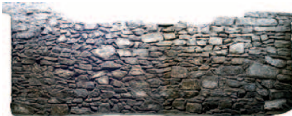
Fig.2: Rectified photograph of south wall Room 4 (before conservation).
